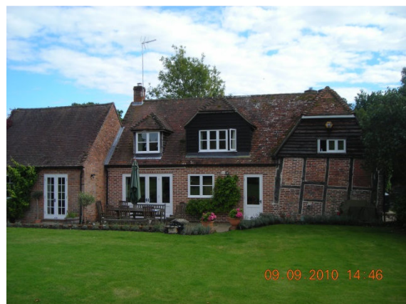
Rear Elevation (close up)
